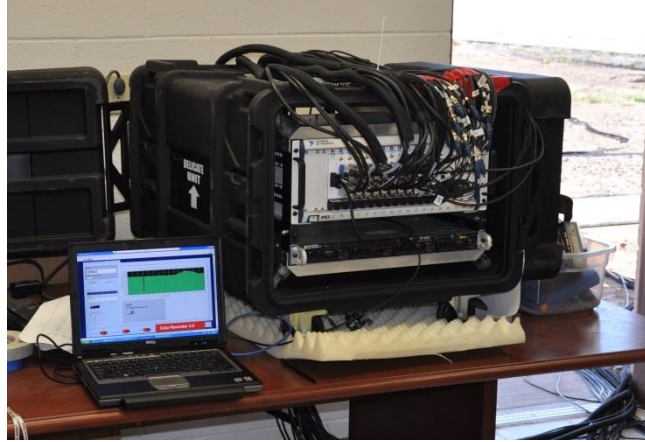
Figure 2.4 Laptop, NI PXI-1045 chassis, and NI 8353 rackmount controller used for data acquisition. The chassis and controller are mounted in a shock mount rack case, and the entire system is in a building located near the run-up pad.
